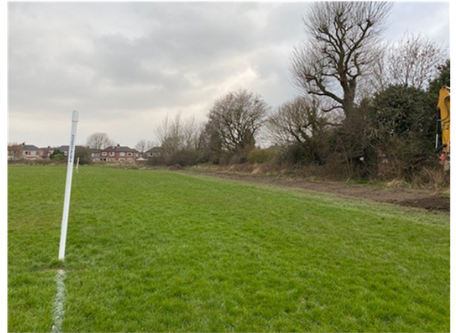
Creation of linear swale looking towards the detention basin
