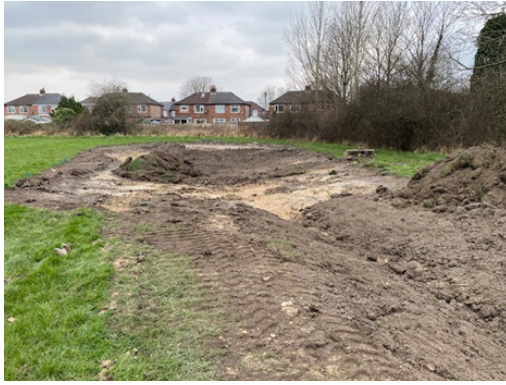
Creation of detention basin
