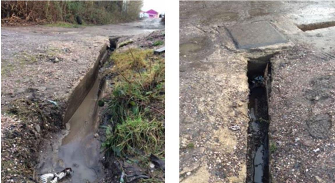
Figure 1: Concrete “drainage channels” discharging surface runoff from vehicle processing yard towards Moston Brook
